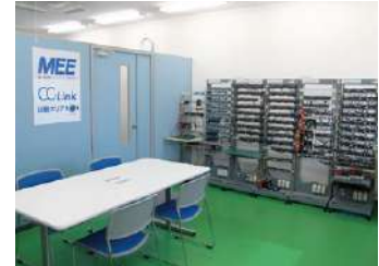
Conformance testing lab
