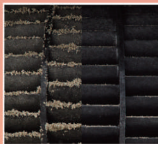
Image after 10 years | Dual Barrier Coating used
